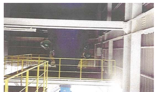
RAW MATERIALS CEMENT Metallic Bunker ALSONS - PHILIPPINE
